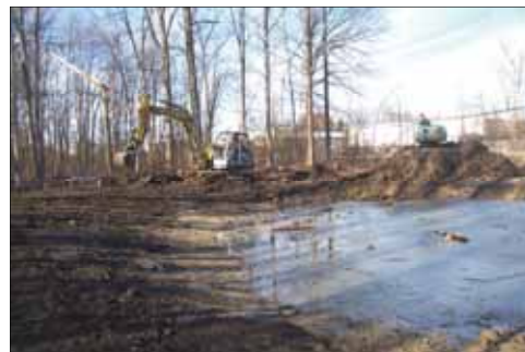
Crawfish Pond excavation
